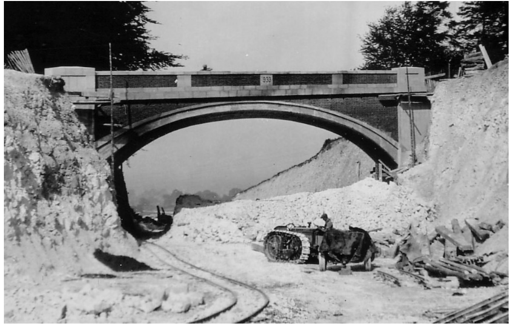
The bridge carrying a private drive across the Hog's Back exit slip road, perhaps suggesting a Lutyens influence. Courtesy of David Rose
